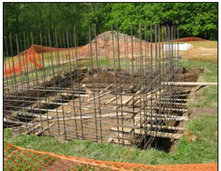
New tower pit, under construction
