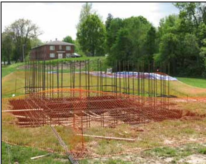
Construction is underway
